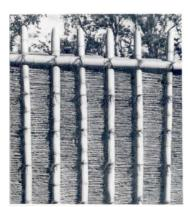
Wall - Protection, barrier, defensive Materials - Bamboo + knotted reeds Connections - man made knots Structure - Grid + rhythmic
