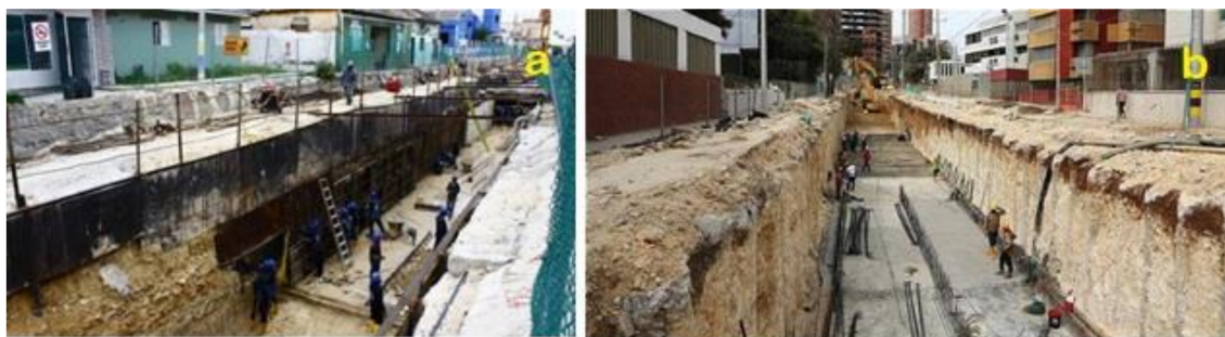
Figure 4. (a,b) Stormwater runoff channel works in the BMA (Source: Mayor’s Office of Barranquilla).
