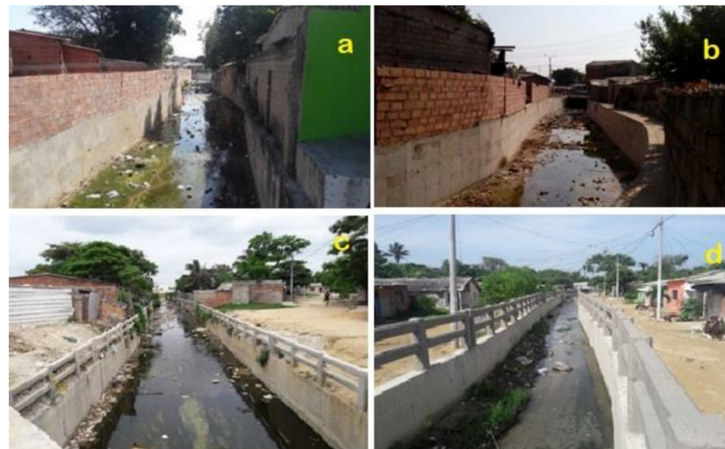
Figure 6. Presence of solid waste in different stormwater runoff channels in BMA. (a) Stormwater runoff channel “El Afan” (Neighborhood San Nicolas); (b) Stormwater runoff channel “Don Diego” (Neighborhood Simon); (c) La Paz Bicentennial stormwater runoff channel; (d) Stormwater runoff channel Village-Sourdis. (Source: Mayor of Barranquilla, 2020).
