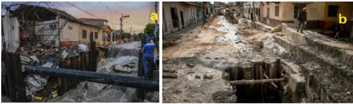
Figure 3. (a) Flooding and its impacts in the HOSPITAL stormwater runoff channel. (b) Canalization works for the HOSPITAL stormwater runoff channel, Street 79 (Source: Mayor’s Office of Barranquilla).
