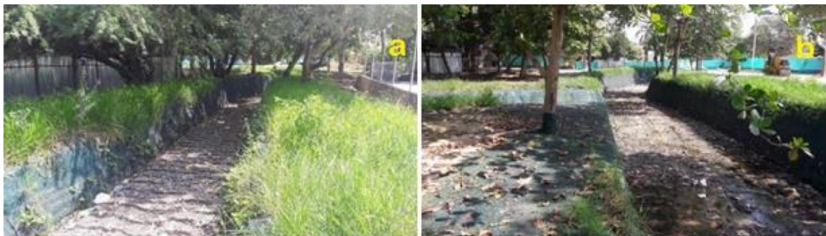
Figure 5. (a,b) Canalization of the Botanical Garden stormwater runoff channel with adaptation measures to the natural environment (Source: Mayor’s Office of Barranquilla).
