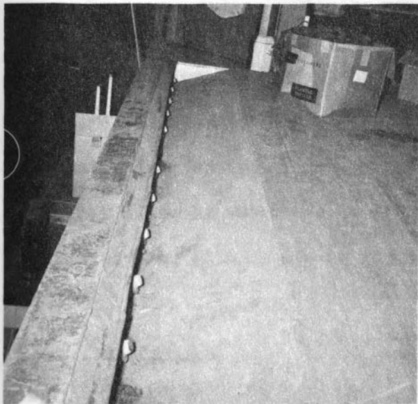
FIGURE 14. Trough in stage apron, 1968.
