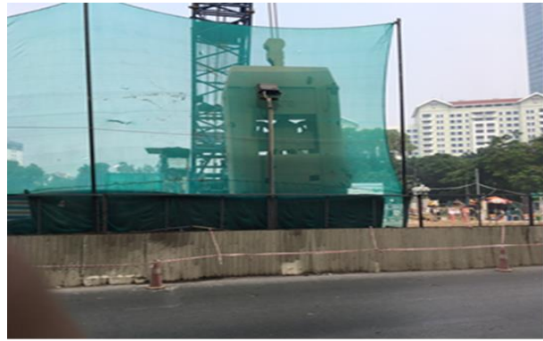
Fig. 6 – Source of vibration – Walls construction machine D-walls
