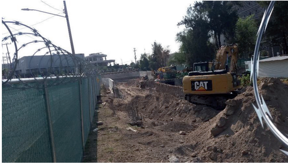
Figure 18. Construction of a dam clothes to Plaza Patria mall, this for contain the rains in the high side of the basin. Source: Jorge Navarro personal files.
