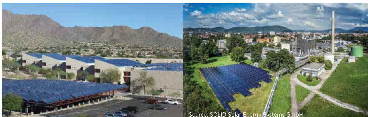
Photograph 7. Solar district cooling plant, Scottsdale, Arizona (United States) (left) and part of the Fernheizwerk collector field, Graz (Austria) (right)
