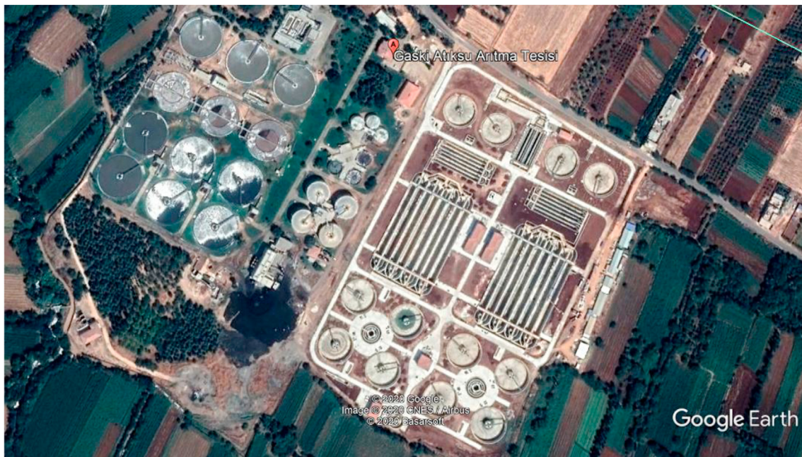
Fig. 17. Satellite view of the GASKI WWTP (Accessed in October 2020).
