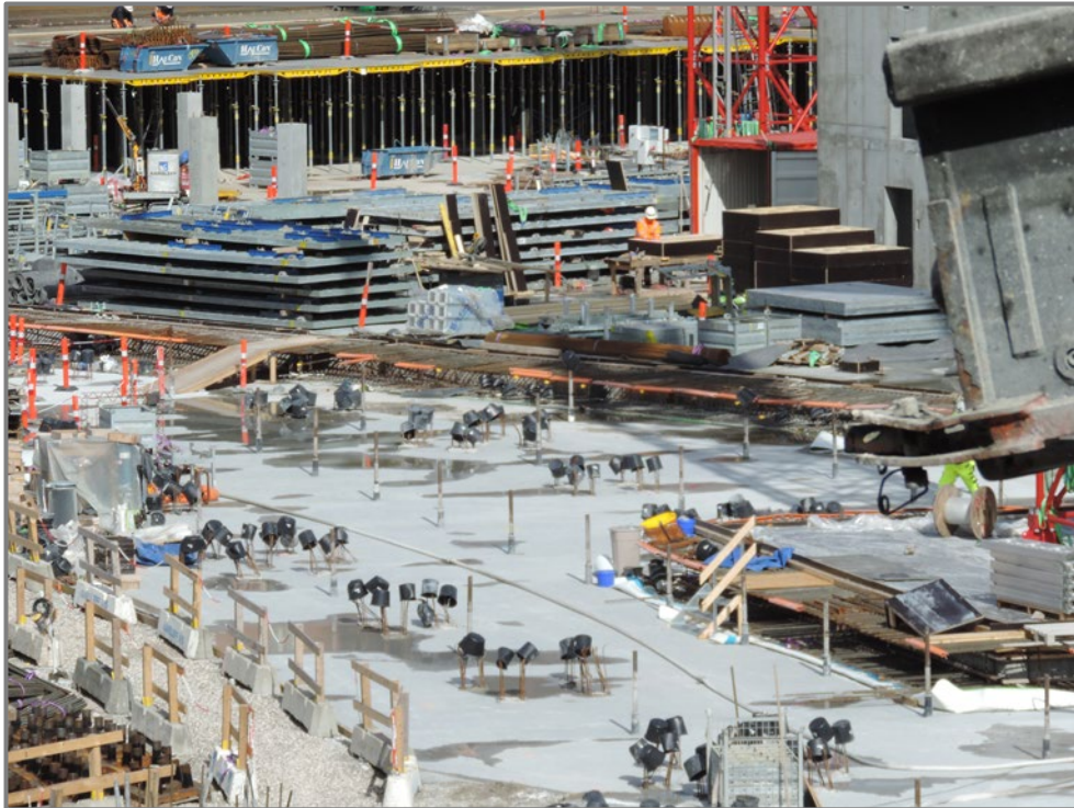
Figure 32. View of the building site 'Postgrunden'.
