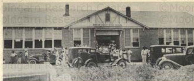
Physical facilities for the Traveling Clinic were various. Sometimes the clinicians had to resort to the dubious shelter and sporadic shade of an accommodating tree while, under more fortunate circumstances, they availed themselves of the better buildings afforded by the communities. The Duncan Center Negro School, in which over one thousand people were served, afforded an excellent site for the clinic.
