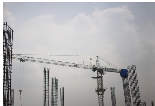
Gambar 2. Tower Crane merk Topkit FO/23B
