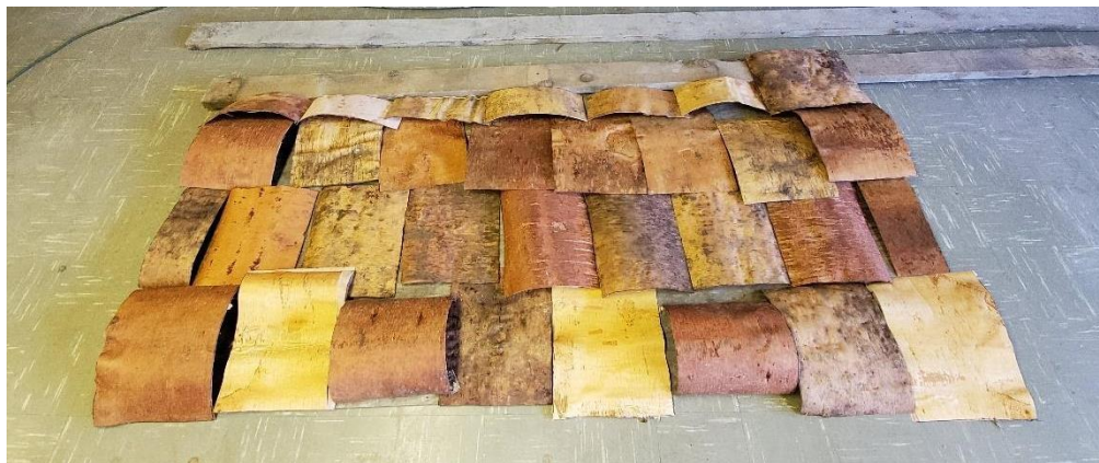
Figure 13: Shingles laid out to determine layout on the roof
