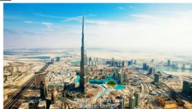
Dubai architecture Source: Google
