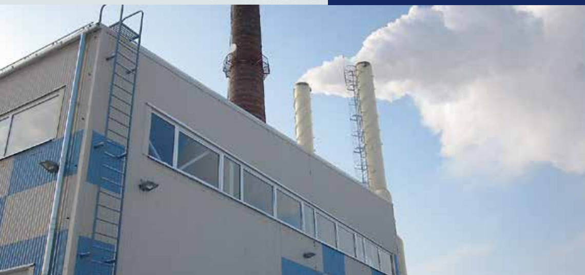
Biomass boiler-house in Tukums
