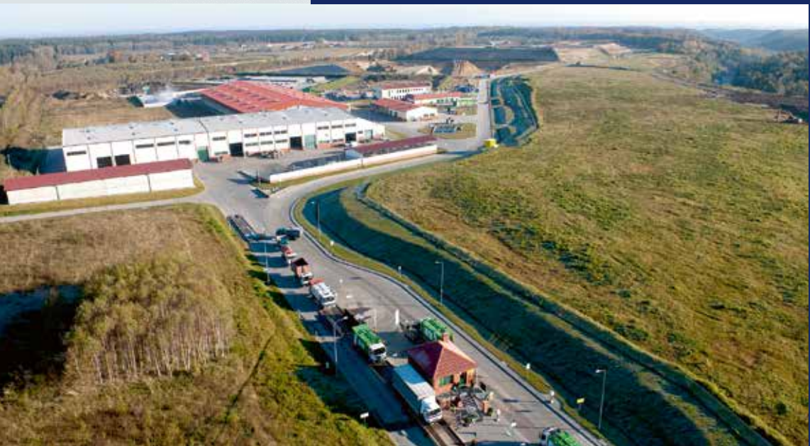
EcoValey - Gdynia recycling and waste utilisation plant
