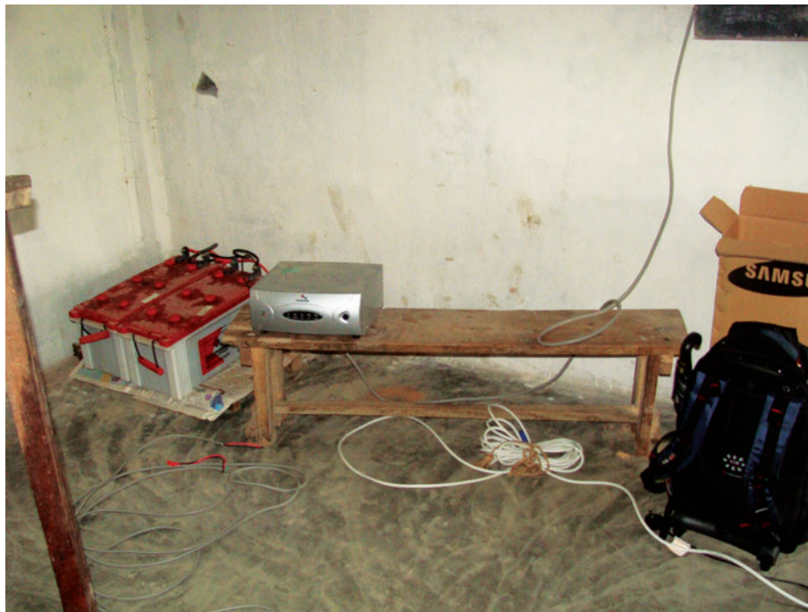
Figure 4. SCR Setup in Progress
