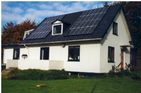
Figure 7 (above). Single family dwelling furnished with 4 kW c-Si PV panels as part of the Solar-300 project (Encon, 2000).
