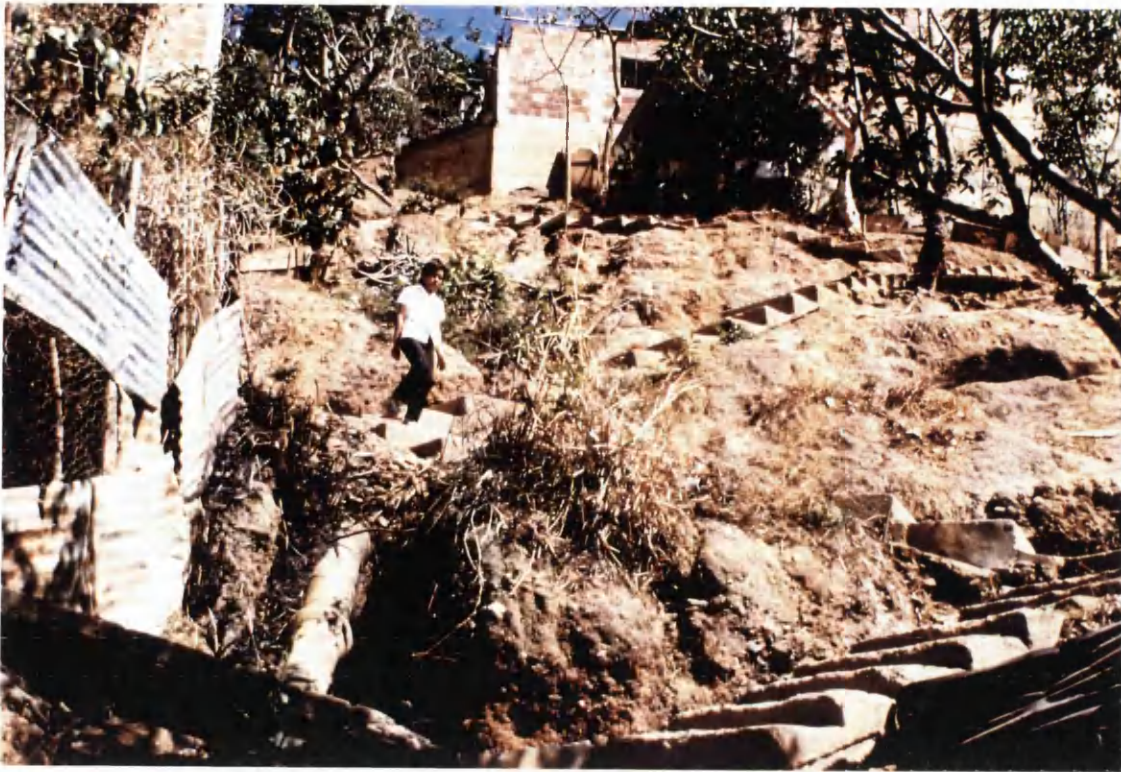
Plate 21: Stairs built up on infill material
