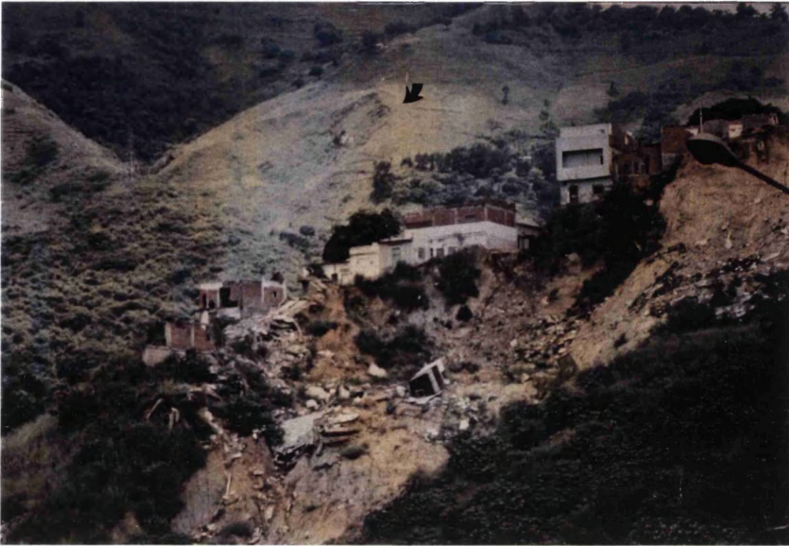
Plate 3: Evidence of slope instability before the settlement process
