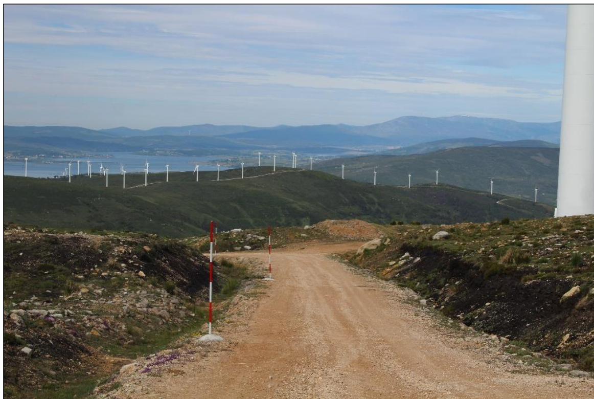
Figure 2.17. Windfarm track construction at Malverde blanket bog in northern Spain (Cantabria).
