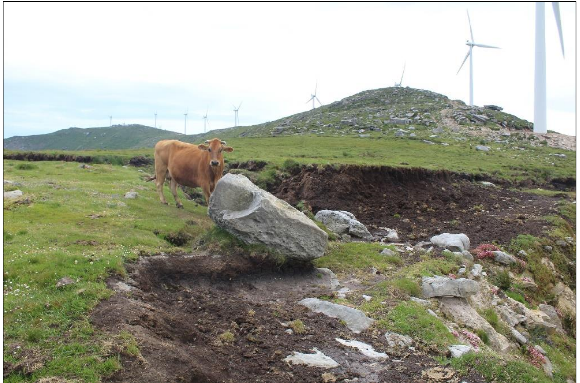
Figure 2.18. Evidence of erosion adjacent to windfarm development in northern Spain (Cantabria).
