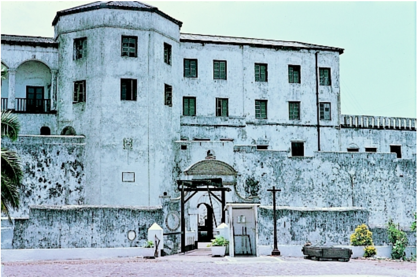
The Castle St. George d'Elmina in the 20th century before the restoration.
