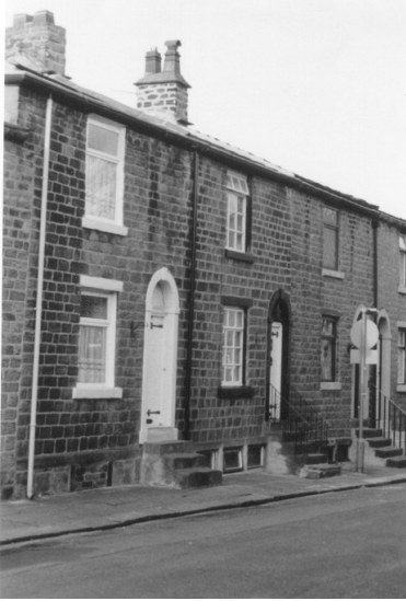
6. Former handloom weavers' cottages with cellar loomshops, West View Place, Blackburn. As in the case of the textile mills, the cottages are of plain appearance, though they have arched doorways with keystones.
