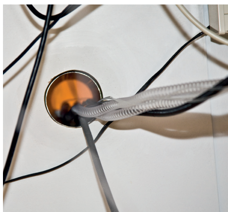
Figure 4. Ventilation hoses, intravenous lines and fibre-optic lead, guided from scanner room to MR control room through a hole in the wall.
