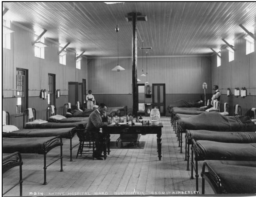
Bultfontein mine compound hospital, 1900s (McGregor Museum Kimberley Photography nr.5354)
