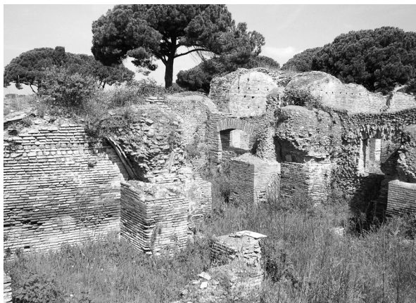
Fig. 5.53 – The walls of the industrial building (IV ii 4) were reinforced with buttresses
