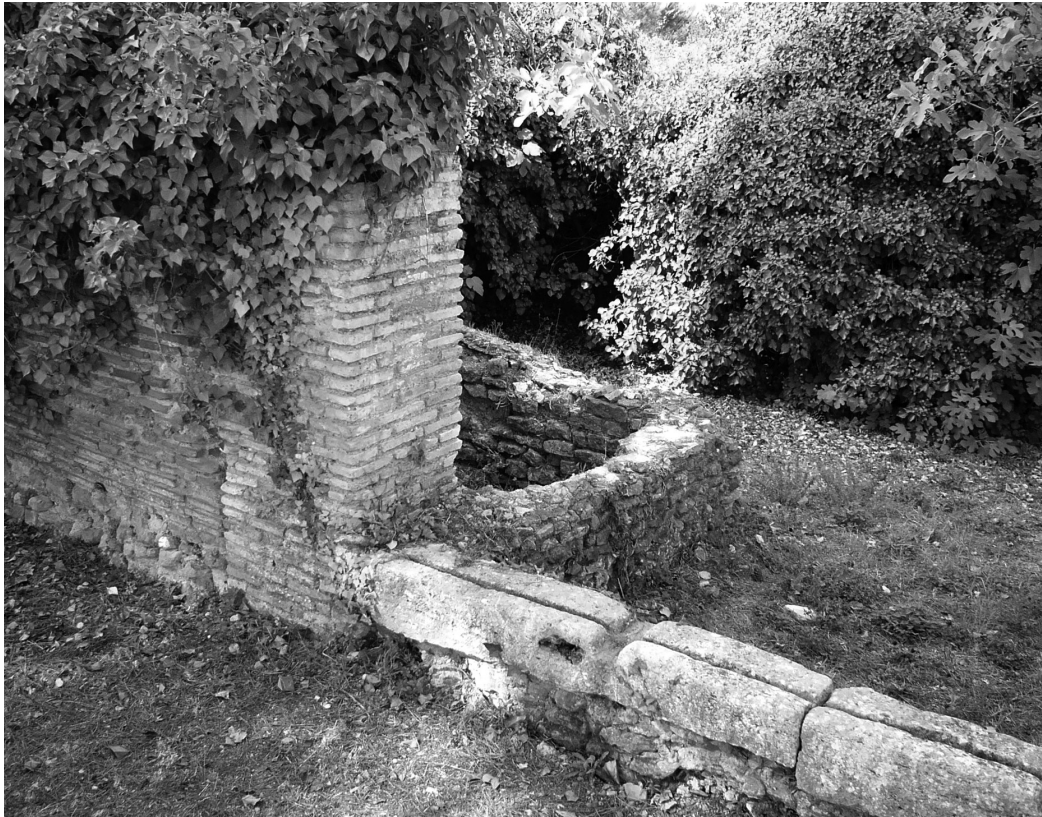
Fig. 5.106 – A travertine threshold marks the entrance to Building IV ii 13 ('Loggia'); the northern corner of the water basin is visible
