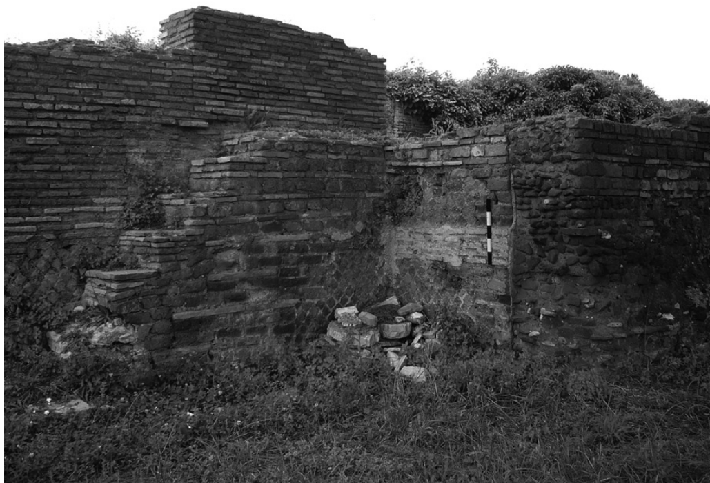
Fig. 5.34 - Stairs and extension built for the construction of the latrine
