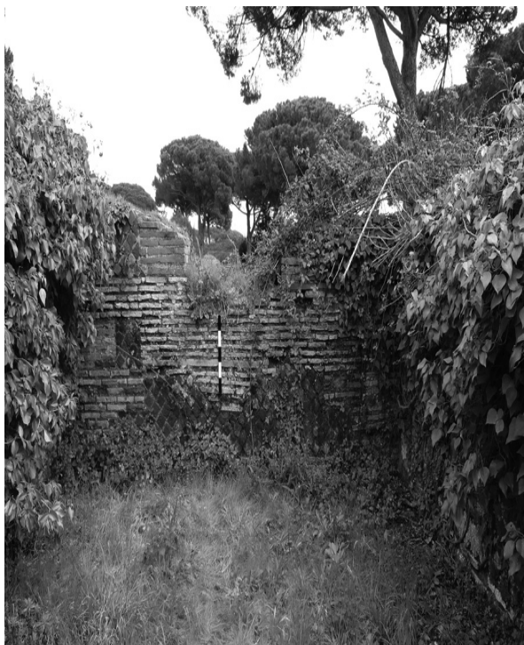
Fig. 5.78 – Building IV ii 8, window in room (8) overlooking the open space to the east
