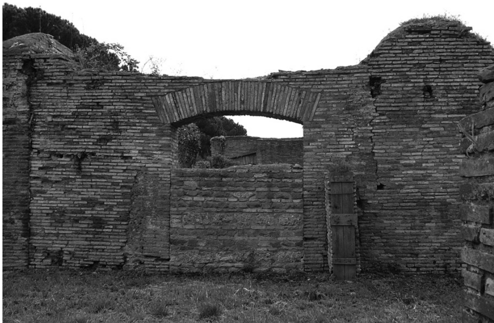
Fig. 5.50 – The entrance leading to the industrial spaces IV ii 3 (030) and IV ii 4 was blocked during a late period of occupation
