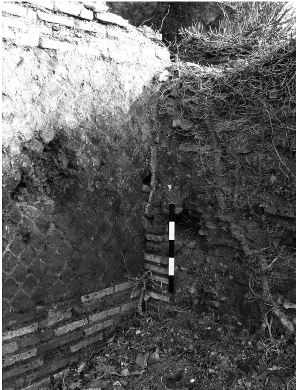
Fig. 5.32 - Painted plaster remains are still visible behind the partition walls
