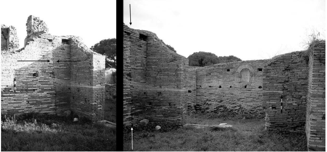
Fig. 5.45 – Room 26: discontinuity is visible in the corners which meet the entrance passage (27)
