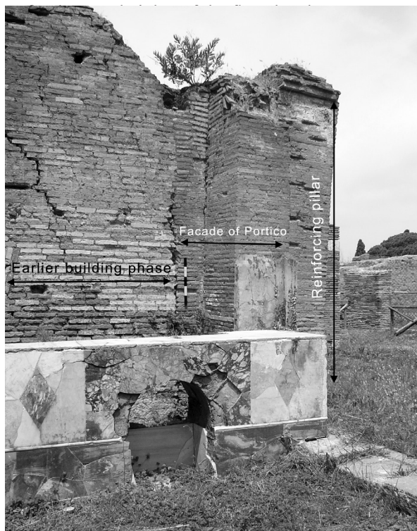
Fig. 5.29 – The facade of the Portico dell'Ercole (IV ii 2) was built against an earlier opus latericium wall
