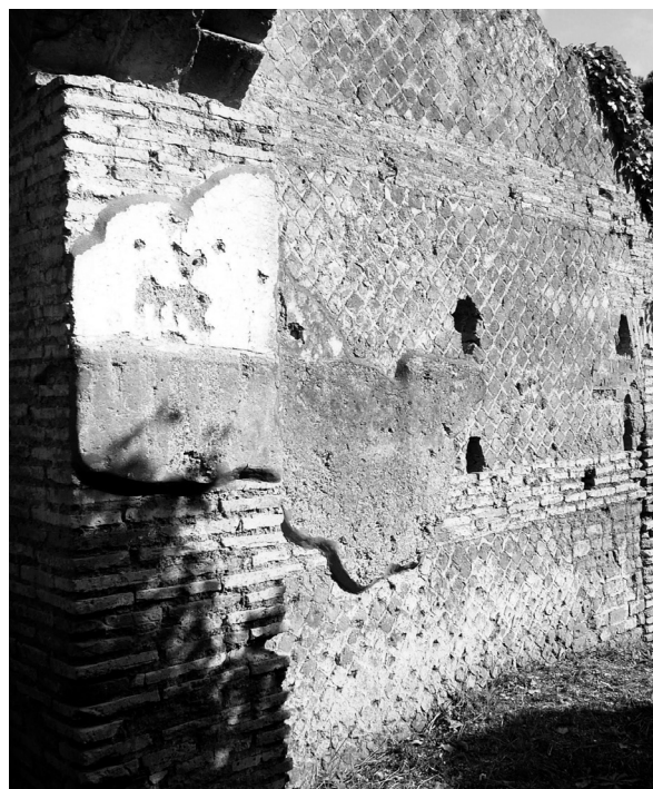
Fig. 5.22 – Painted plaster remains in northern changing room ( apodyterium [07])
