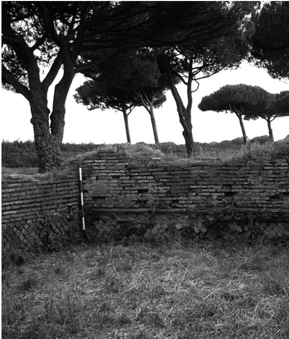
Fig. 5.87 – Southern wall (room 6) which confines Building IV ii 10 against the open space to the south; remains of floor levels are indicated by a course of bipedales and traces of mosaics preserved in the corners
