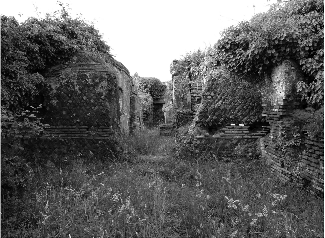
Fig. 5.60 – Opus reticulatum structures of the adjacent Building IV ii 12
