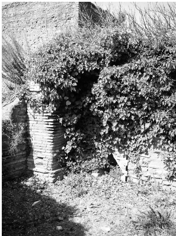
Fig. 5.107 – North-western corner within the 'Loggia' with a water channel constructed from bipedales
