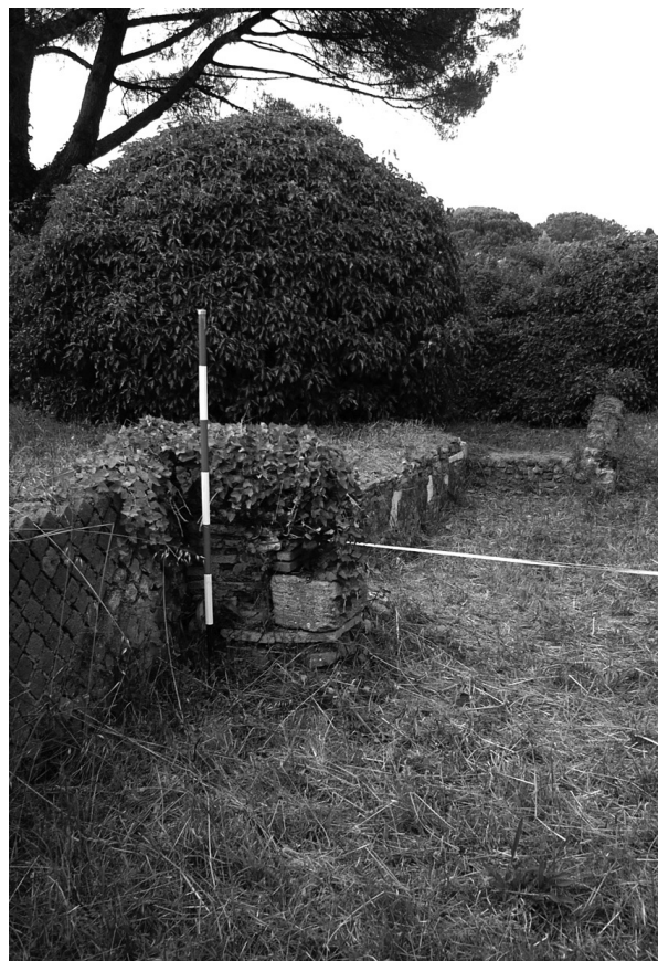
Fig. 5.89 – Building IV ii 10, higher floor levels are only preserved in the western rooms 1 and 4
