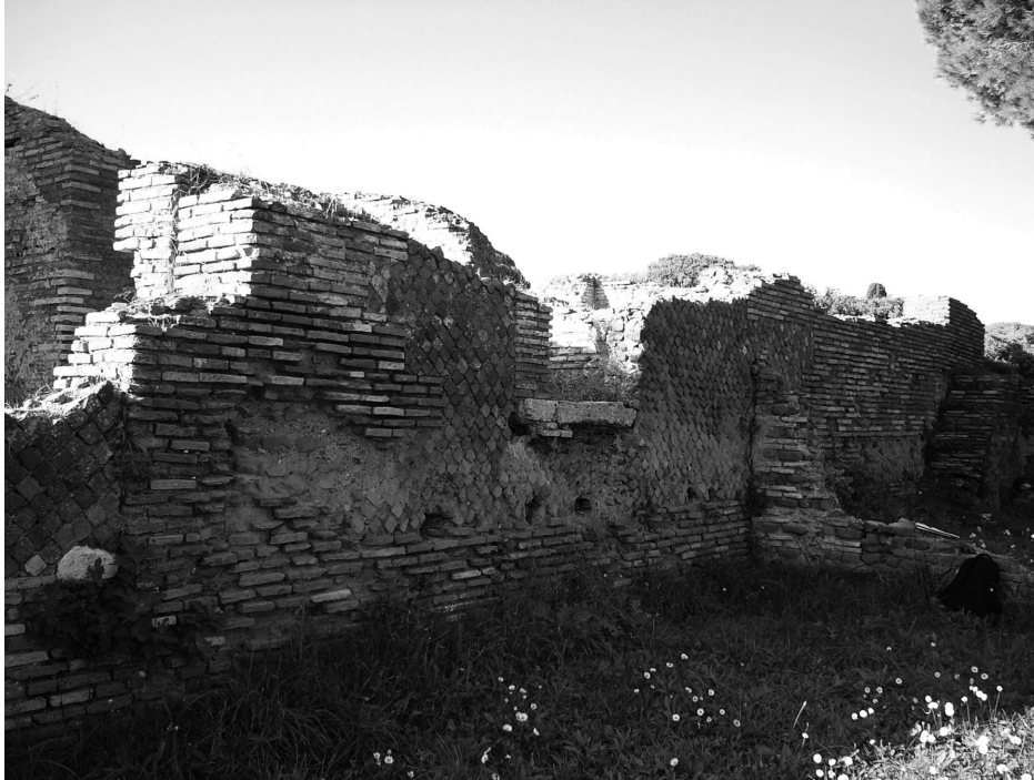
Fig. 5.33 - Connecting door between baths and Campo; the difference in height was probably overcome by wooden stairs; the beam holes could be connected to a ramp or some other temporary construction
