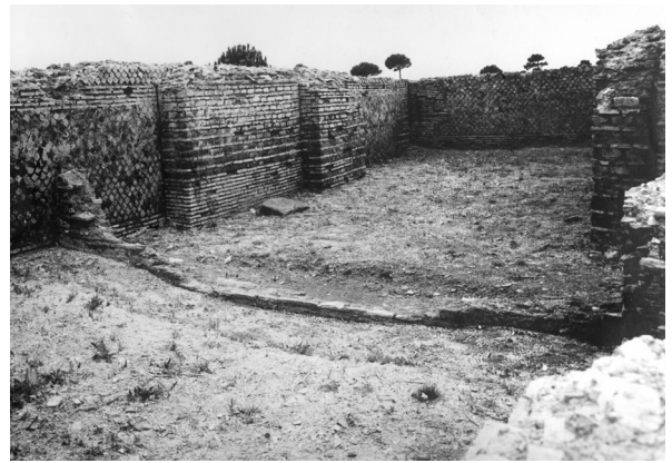
Fig. 5.74 – Hall (06/07) in the south-eastern corner, partition wall is clearly visible in the foreground (Scavi di Ostia, Archivio Fotografico, ref. 3764)
