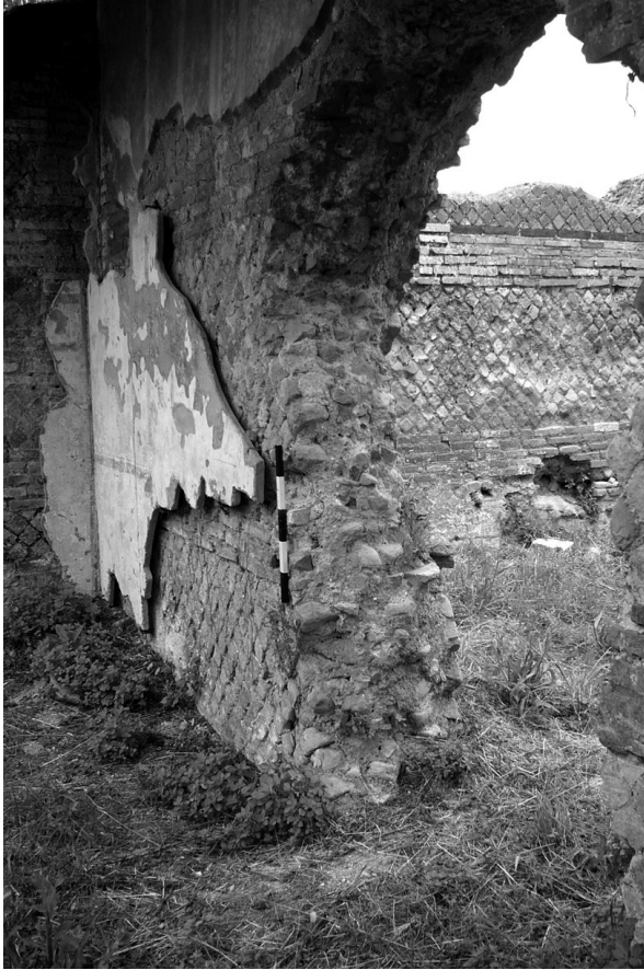
Fig. 5.111 – Door openings were broken into the opus reticulatum wall to interconnect all tabernae
