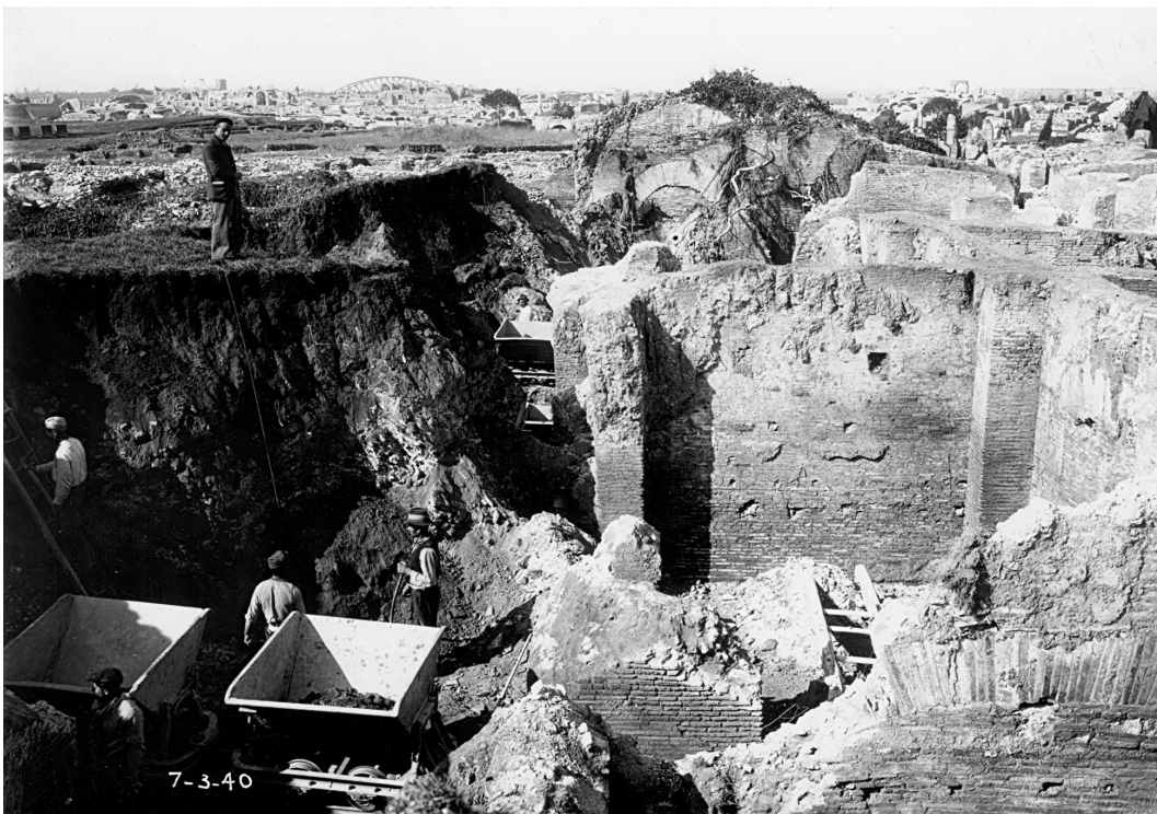
Fig. 5.37 – Excavation in process: the courtyard is still under excavation, dated March 7th 1940 (Scavi di Ostia, Archivio Fotografico, ref. B 2901)
