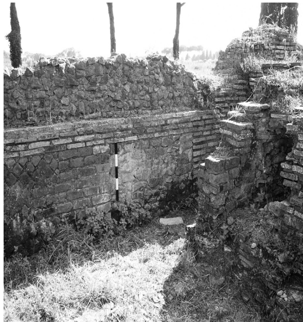
Fig. 5.96 – A former door opening in the mithraeum 's southern wall betrays an earlier connection to the open space in the south
