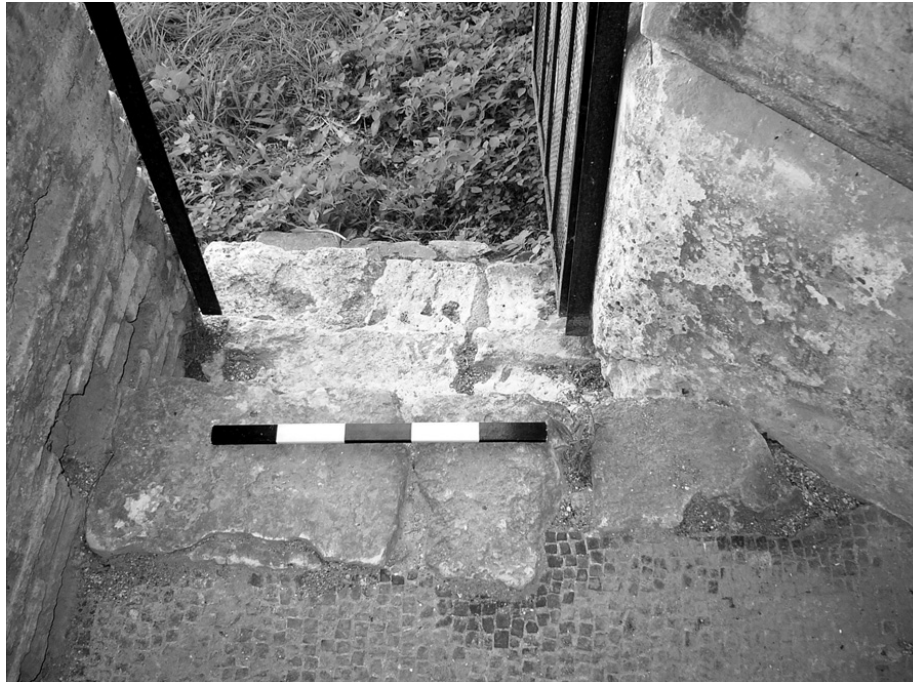
Fig. 5.63 – Difference in height between the Caupona's floor levels (corridor 06) and the rear courtyard (07)
