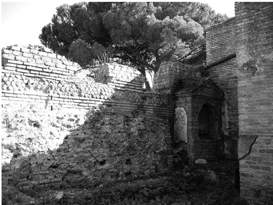
Fig. 5.65 – The aedicula-type niche located in the south-eastern corner of the Caupona's courtyard; walled benches were placed against a crude wall; the latter was built against the opus reticulatum (brick) wall of building IV ii 14
