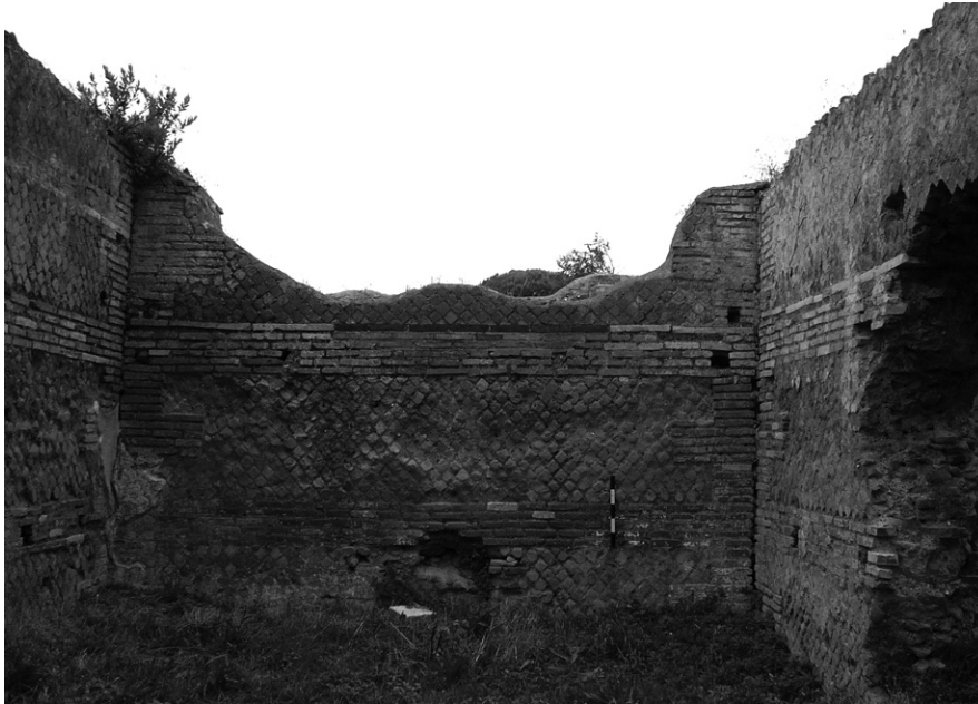
Fig. 5.110 – Opus reticulatum with regular fields of reticulatum; corners are reinforced with quoining in opus latericium ; a former door opening betrays a link to the neighbouring building to the north
