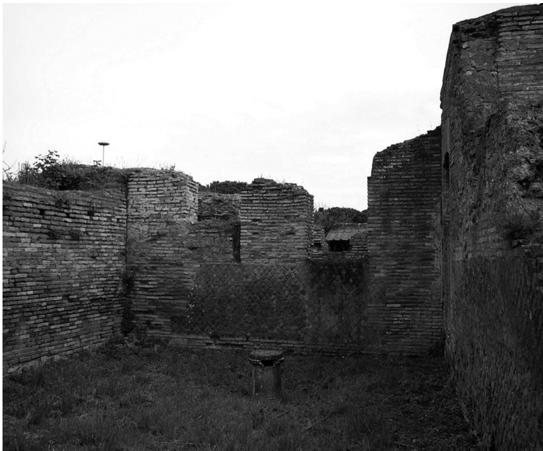
Fig. 5.67 – Room 16, the well head communicates through a shaft to the chamber below which can be accessed from courtyard (07)
