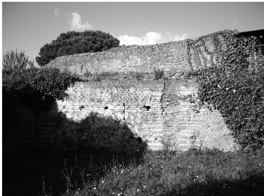
Fig. 5.71 – Caseggiato IV ii 7, northern wall abutting the Caupona del Pavone (IV ii 6); walling technique employs quoining with tufa and brick; traces of a former perpendicular division are still visible
