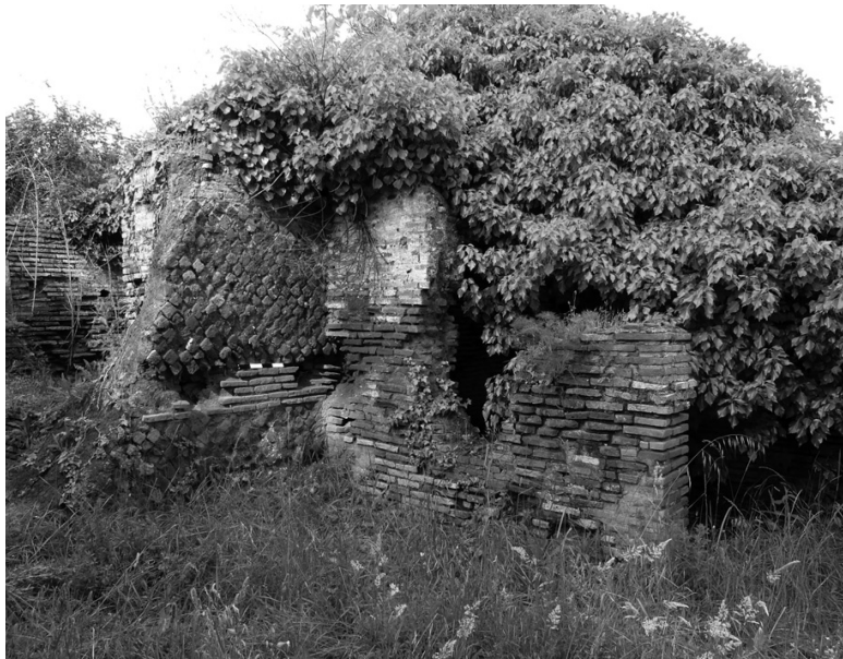
Fig. 5.102 – Building IV ii 12: partition wall between room 02 and the room behind the eastern staircase (03), the wall was built against the earlier opus reticulatum (brick) wall
