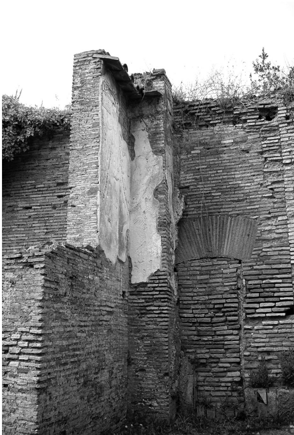
Fig. 5.27 – Walled-up door connecting room 06 to the space west of the baths, presumably walled up when the outside space was occupied by the water cistern
