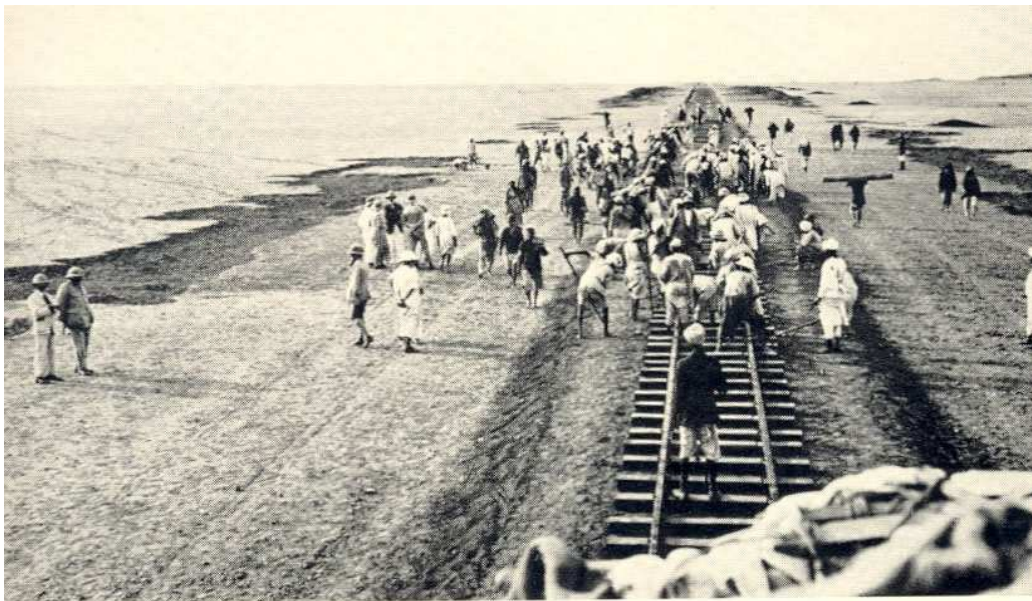
Picture 3: Railway construction Source: Hill, Sudan transport, plate 4
