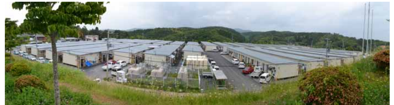
Temporary Housing Area
