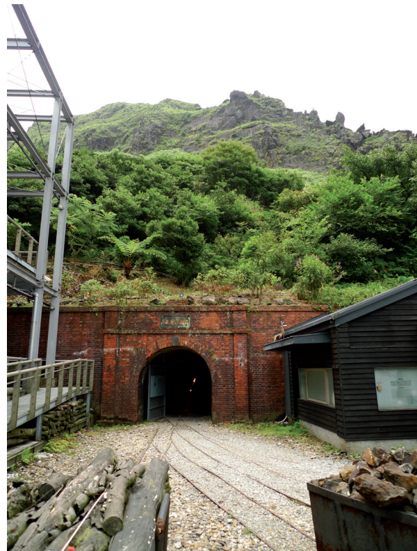
Fig. 3.1.7 The Benshan Fifth Tunnel. Photo was taken by the author.
