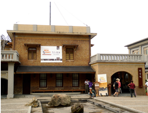
Fig. 3.2.8 The Gold Refinery Building. Photo was taken by the author.
