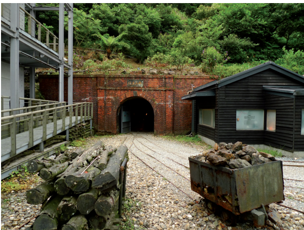
Fig. 3.2.4 The Benshan Fifth Tunnel. Photo was taken by the author.
