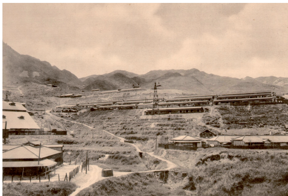
Fig. 3.1.3 The long residences of miners in 1914. Courtesy of National Taiwan University Library.
