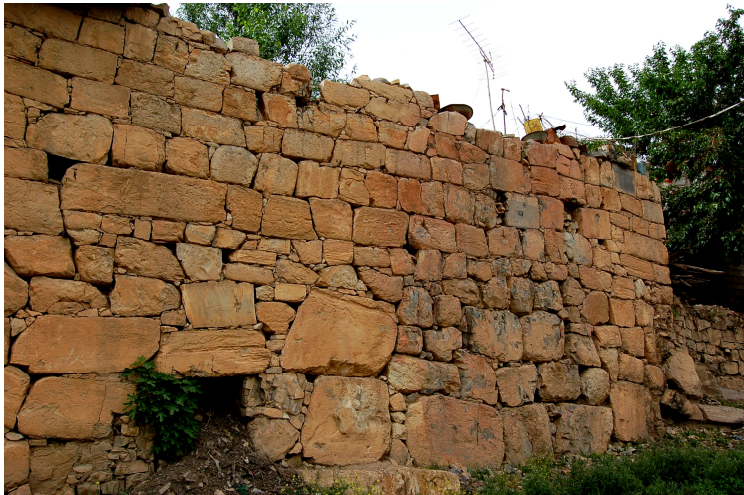
16a) An old cyclopean stone wall built on a still older portion. The wall is at the foot of the citadel and at present forms one of the walls of a dwelling house in Bētwater. Photo by the author.
