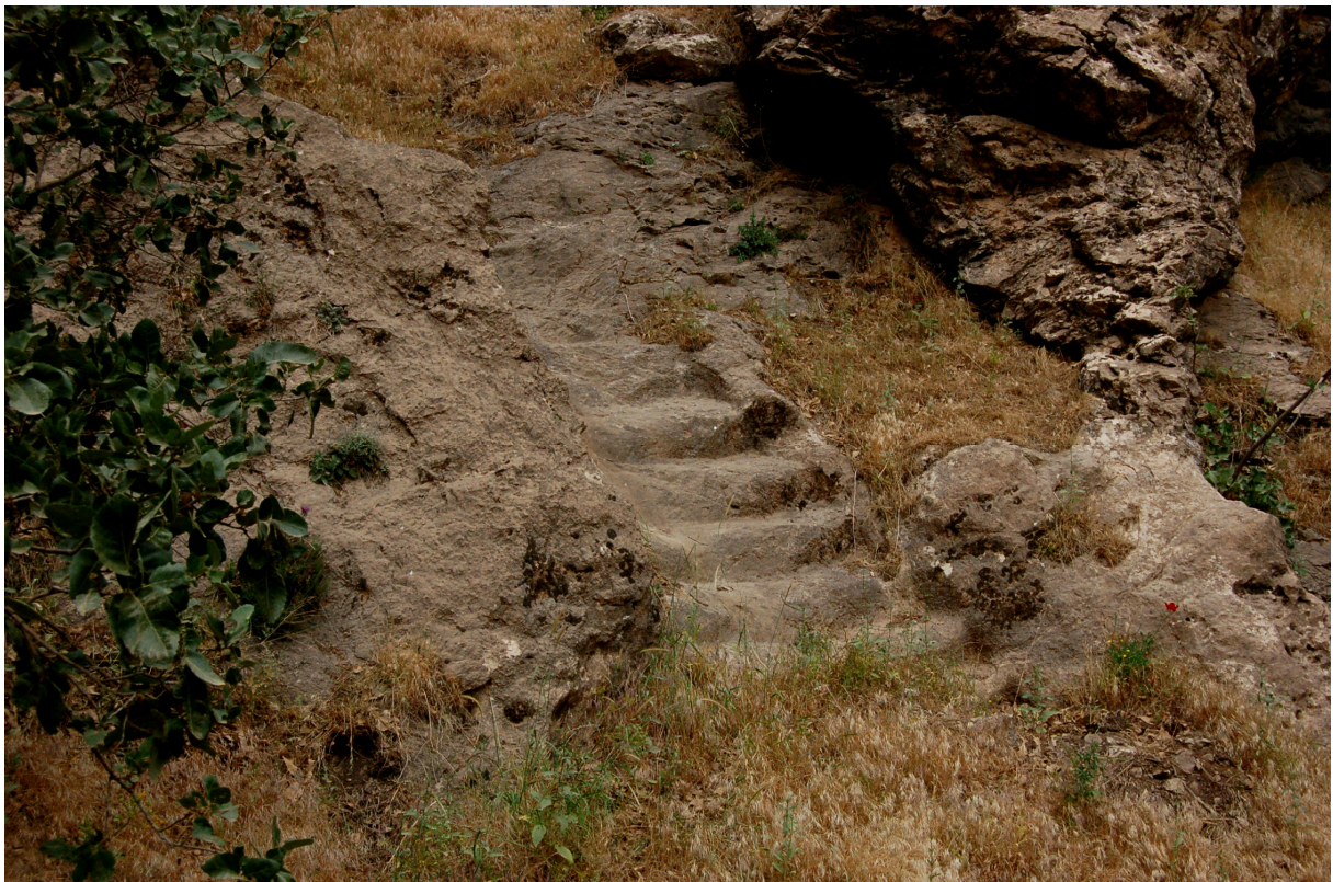
22b) The second staircase to the west of the lower passage (Stc. no. 2). Photo by the author.
