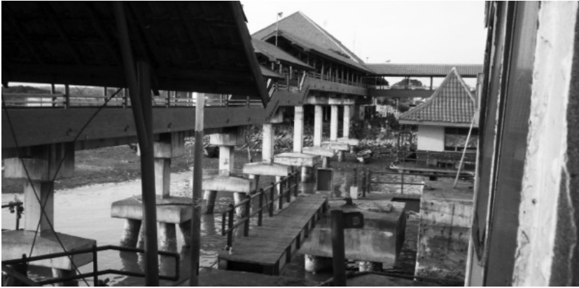
Figure 11: Kamal seaport in the Bangkalan regency that connects Madura and Java
