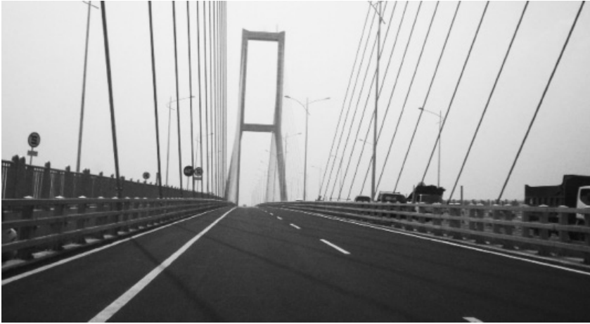
Figure 7: Crossing the Madura Strait via the Suramadu Bridge
