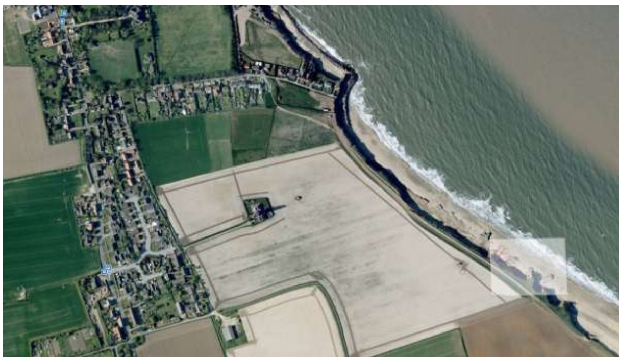
Figure 15 - Excavation area in relation to Happisburgh town.
