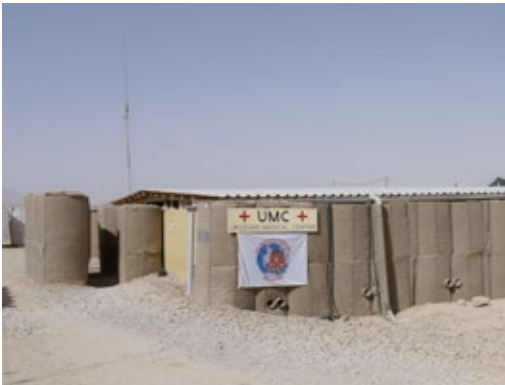
Figure 1. The Dutch role 2 Medical Treatment Facility in Uruzgan, Afghanistan, reinforced by a ballistic protection wall (Hesco-Wall).
