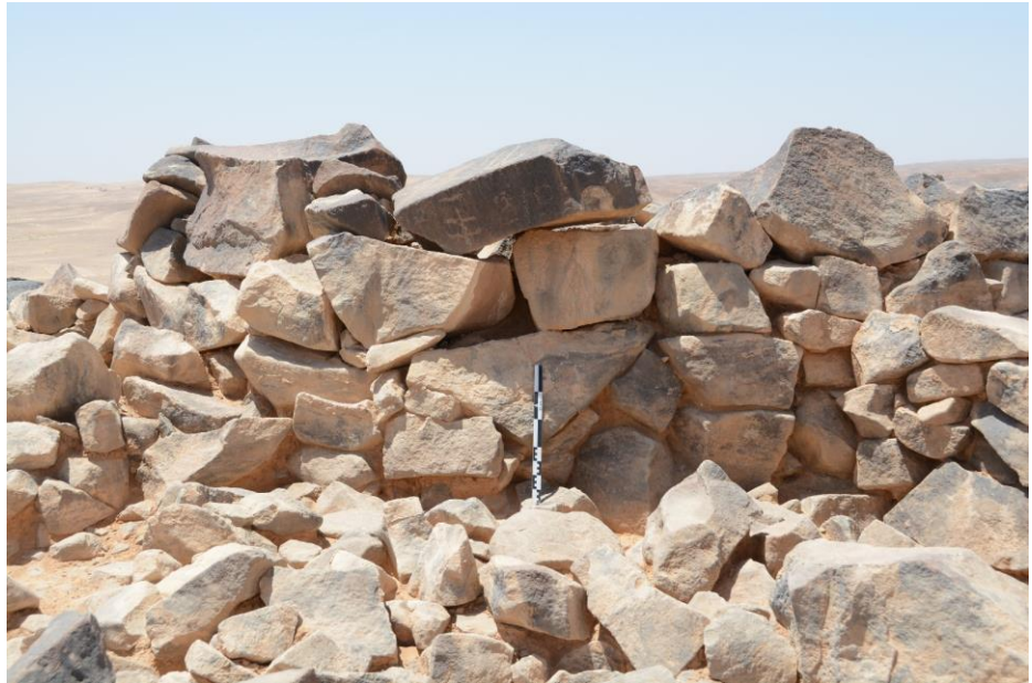
Figure 5.36: Façade of Structure 13 (QR-2). Scale is 50 cm, photo by P. Akkermans.
