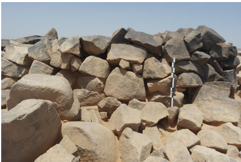
Figure 5.46: Façade D of Structure 23 (QR-148) as exposed through excavations. Scale is 50 cm, photo by author.
