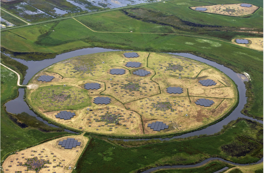
Figure 1.6.: The innermost stations of LOFAR. The stations located in the central circular region, a terp , are known as the superterp stations. The LBA and HBA dipoles can be identified by their arrangement in the field. The LBA dipoles are distributed in a non-uniform way, while the HBA dipoles are arranged into compact groups.
