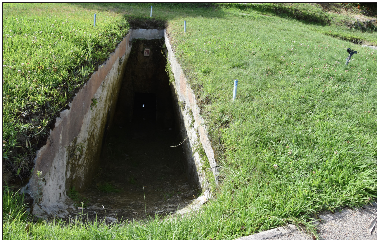
Figure 4.3.16. VT28 entrance, facing south-southeast.
