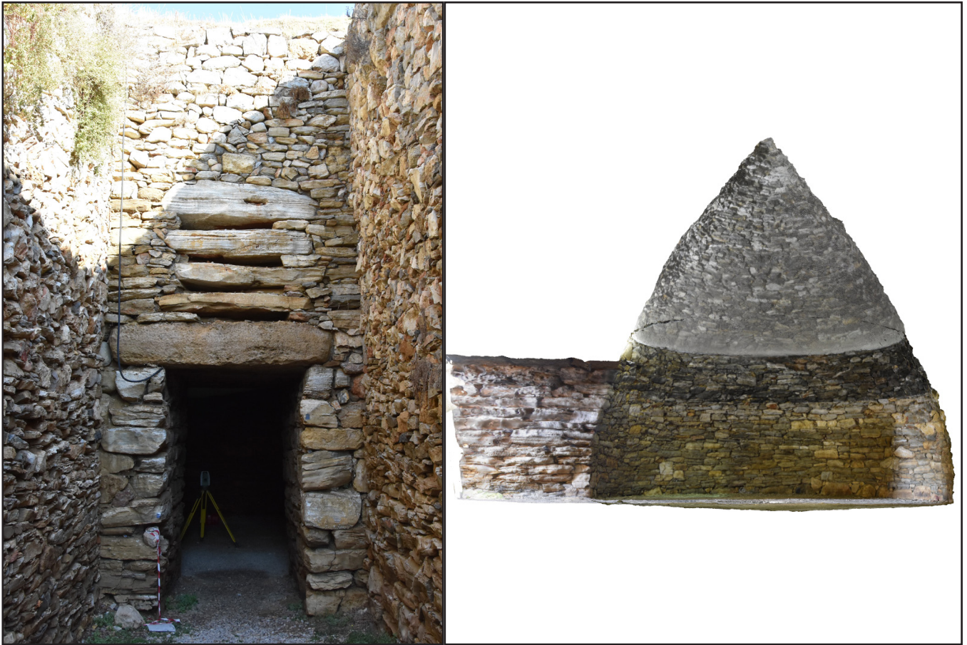
Figure 3.1. Trabeated and corbelled spanning at the Menidi tholos .
