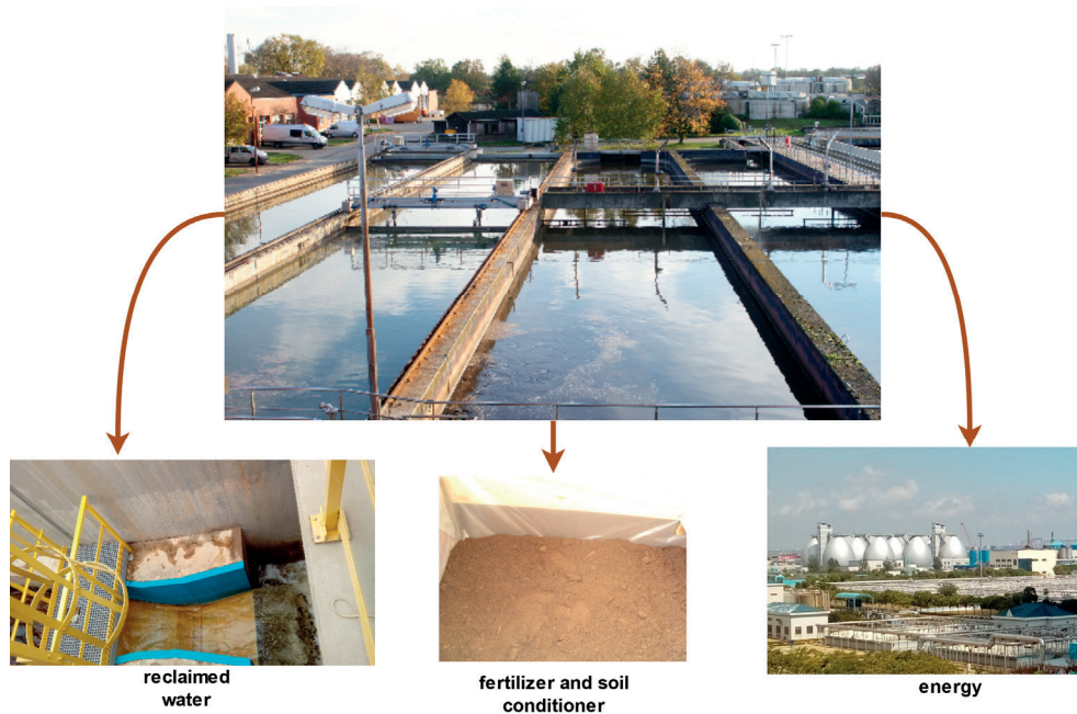
Fig. 12. Illustration of a water resource recovery facility (biorefinery) with some resource recovery practices.
