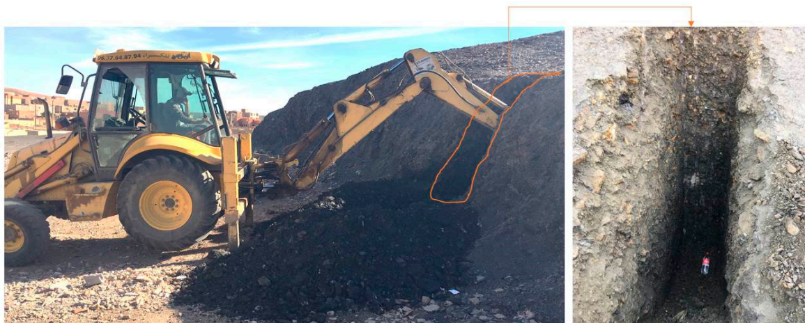
Figure 2. Coal mine waste rocks (CMWR) sampling with a loader machine.
