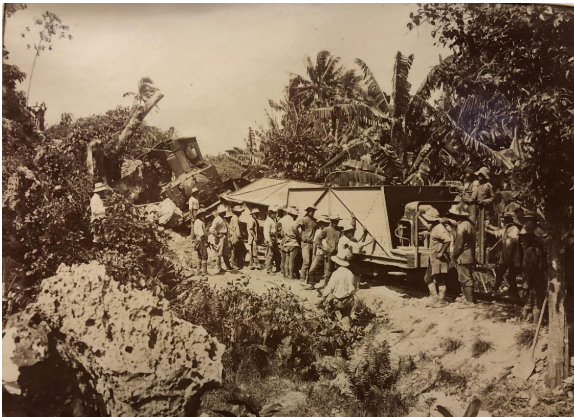
Figure 3.6: Derailment of 30 October 1914, Makatea. Source: Alexander Turnbull Library, PA1-q-156.
