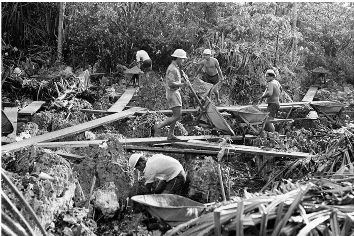
Figure 6.2: At the Diggings ( les travaux ).
