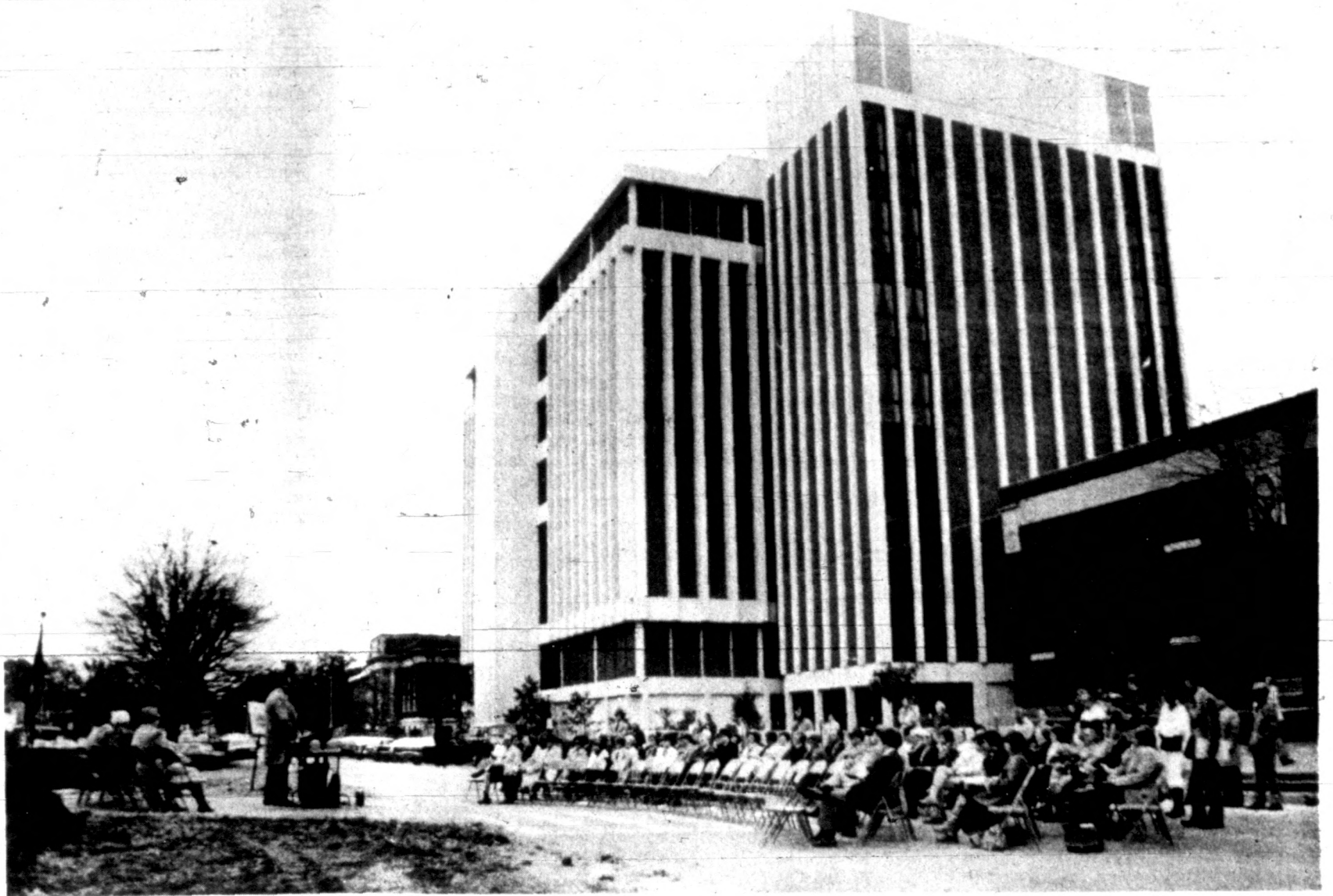
NEW LIBRARY CONSTRUCTION —Several state, city, and county officials were present at the groundbreaking for a project to convert the Waterfield
