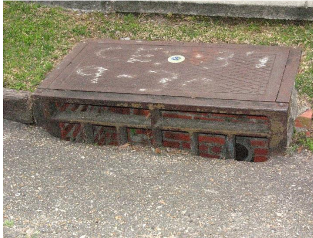
Storm Drain (rating 1) open/un-blocked
