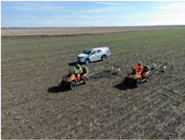
Photo 5: Use of MAGNEX 120LW device on Demining and Technical Survey Project (UXO risk reduction) in the areas of construction of the main gas pipeline from the border with Bulgaria (near Zaječar) to the border with Hungary (near Horgoš).
