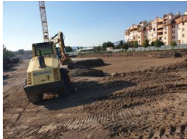
Fig 1: Armored excavator used on ERW clearance project in Niš
