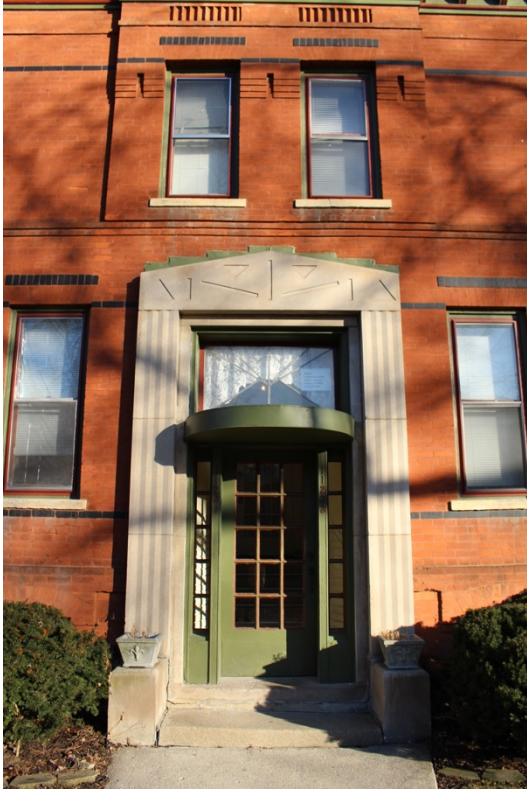
Figure 4.40. Moderne-style door surround added to 11233 Champlain Avenue. Photo S. Scarlett.
