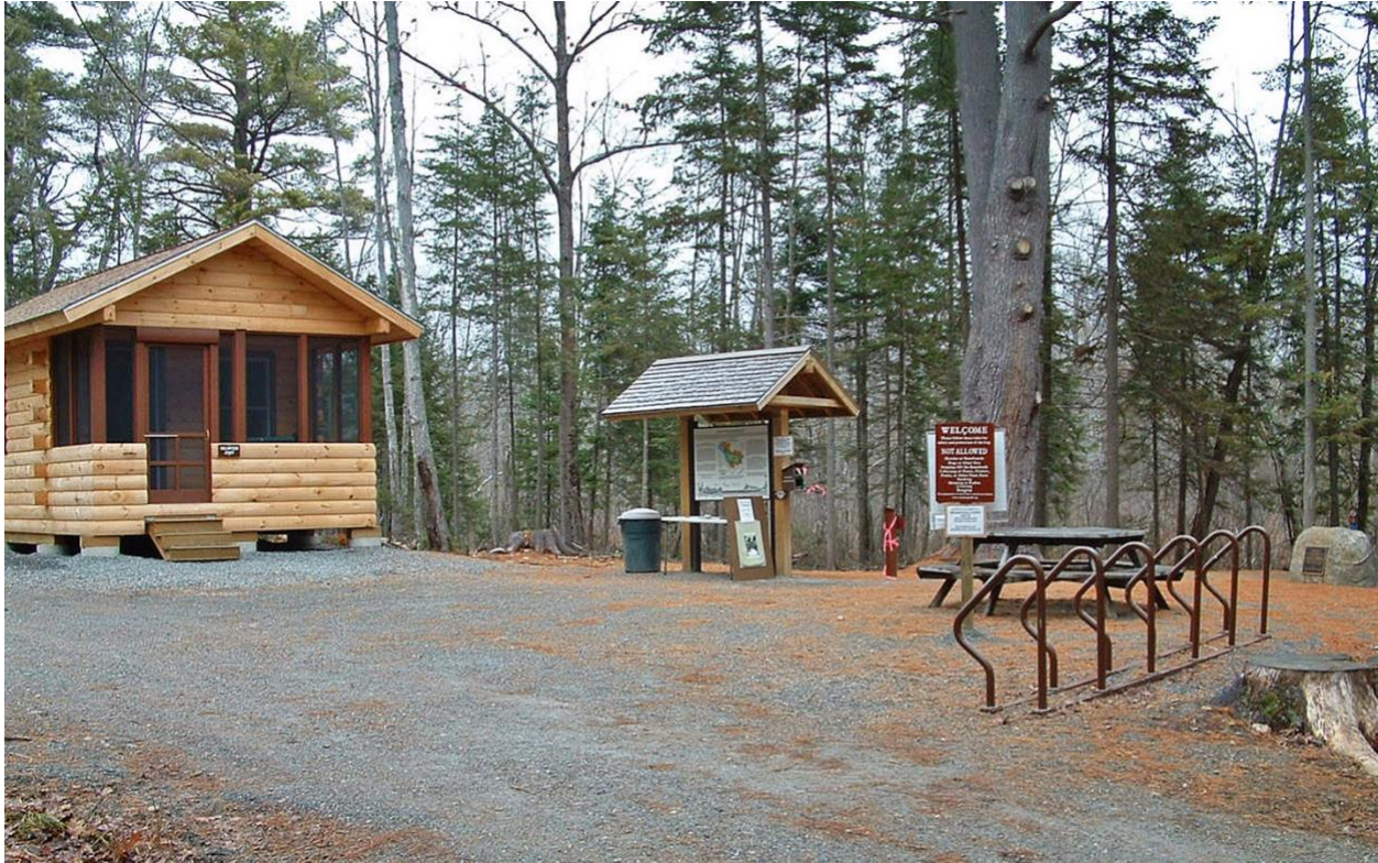
Fig. 14. Information area in November 2004. Facilities from left to right and references to more detailed illustrations: (1) cabin (Fig. 35), (2) kiosk (Fig. 27) with introductory sign (Fig. 24) and visitor registration box, trash container, display table, and event announcement signs, (3) money pipe (for donations), (4) rules sign, (5) picnic table, (6) bike rack, and (7) boulder with National Natural Landmark plaque (Fig. 25). Only the beginning of the short path to the boardwalk entrance can be seen (left of the boulder). The path runs from left to right and downslope behind the boulder. Ronald B. Davis photo.
