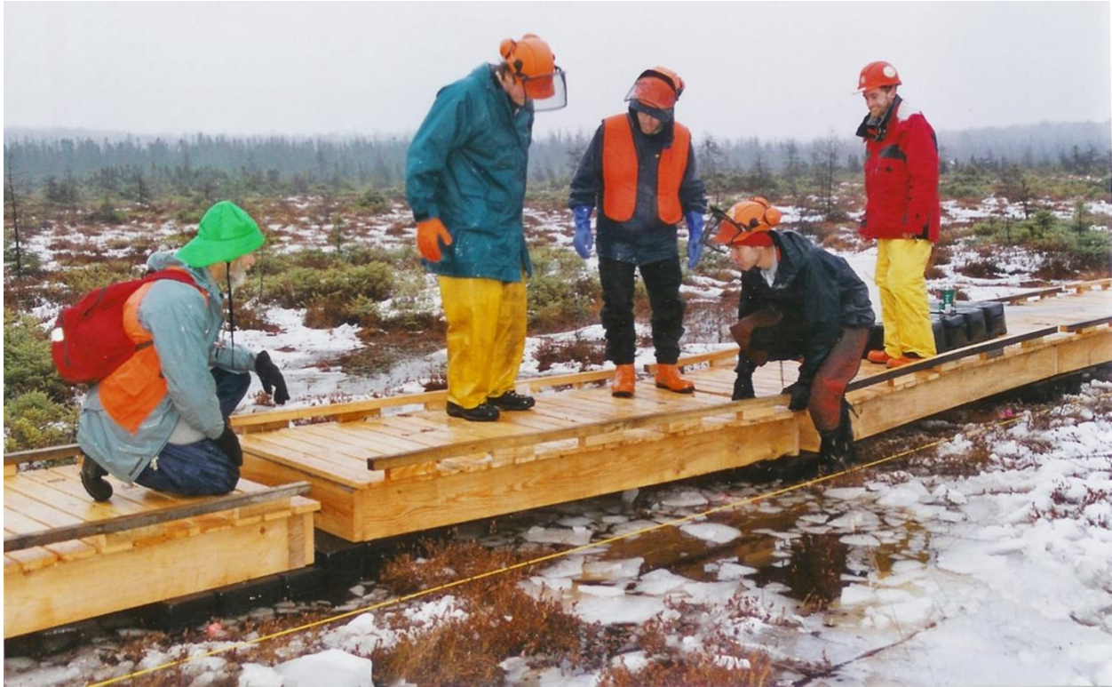
Fig. 22. Adjusting the final or 509 th placed section shortly after the two arms of the boardwalk loop were joined by it at the middle of the open bog at 2 PM on 22 November 2002. It was a cold, wet and dreary day, but we still were all warmed by the glow of the “drive the golden spike” occasion moments before. The remaining gap of about a 1 ft (~0.3 m) would be easy to bridge when work resumed in spring 2003. Author Ron Davis in green hat observes the four MCC leaders. Photographer unknown.
