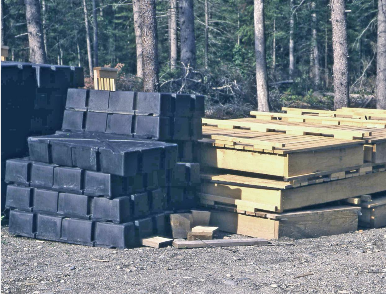
Fig. 18. Floats and sections stockpiled at assembly site. Floats are 4 x 2 x 0.67 ft (~1.2 x 0.6 x 0.2 m). Ronald B. Davis photo.
