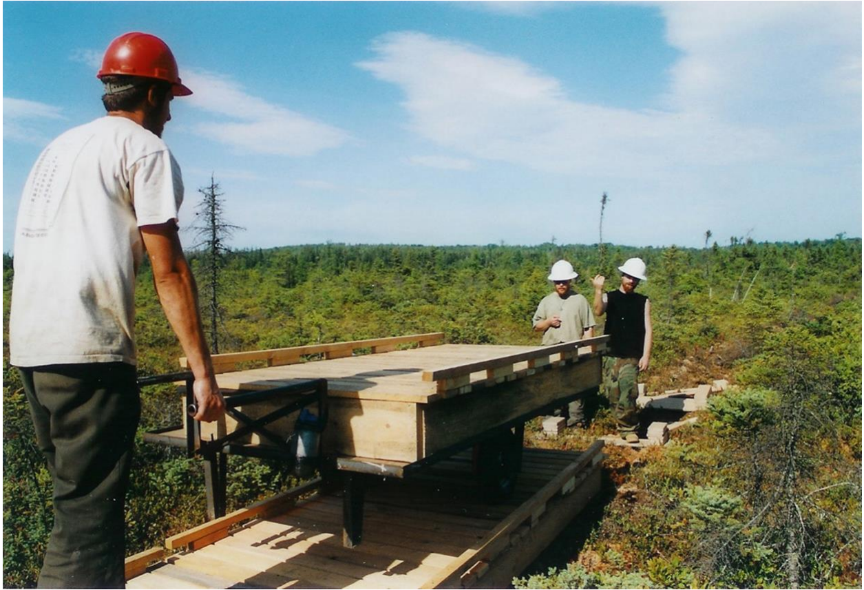
Fig. 19. Arriving with a section at end of incomplete boardwalk. The pair of MCC members in the bog have prepared footings for supporting the arrived section. Ron Lisnet UM photo.
