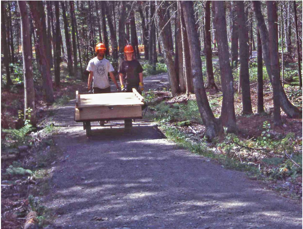
Fig. 13. Transporting a boardwalk section on a special cart along the trail from the assembly site to the incomplete boardwalk. Ronald B. Davis photo.
