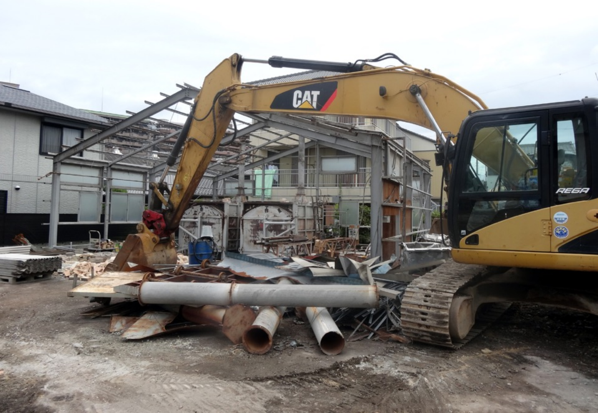
Demolition of the Jinno Porcelain Factory, September 2016.
