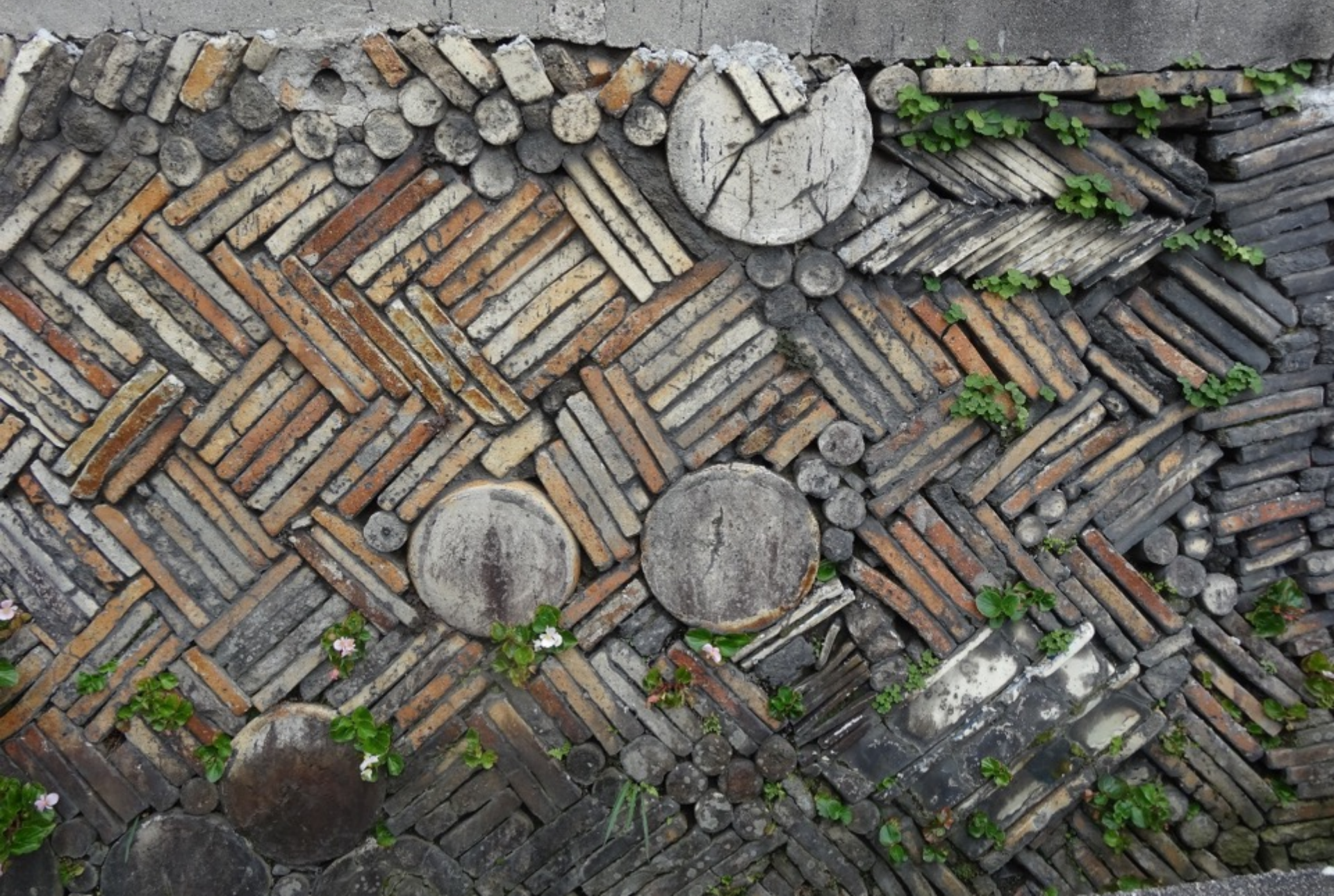
Kiln furniture (supports, sagars & shelves) incorporated into revetments around Seto, especially on the 'The Path of the Kiln Fence' (窯垣の小径).
