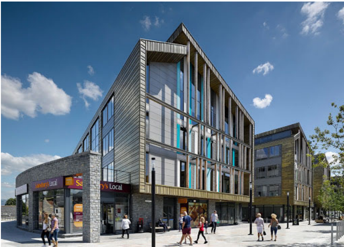
Figure 4.1: External view of the public office building
