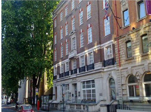
Figure 4.26: External view of the university office building
