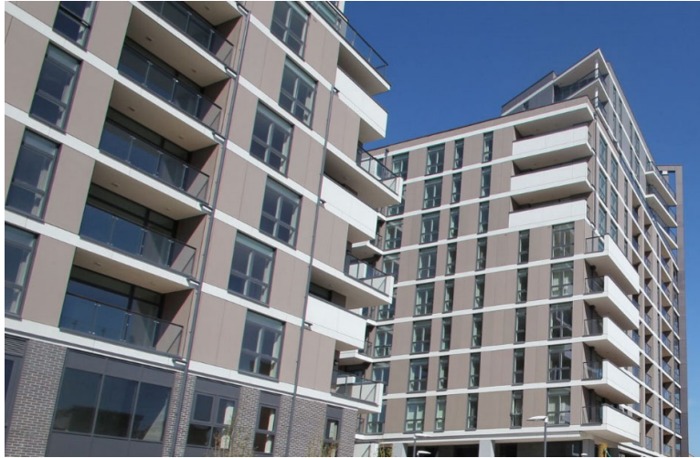
Figure 4.20: External view of the building
