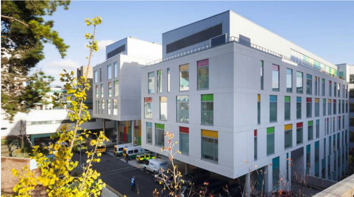
Figure 4.14: External view of the building
