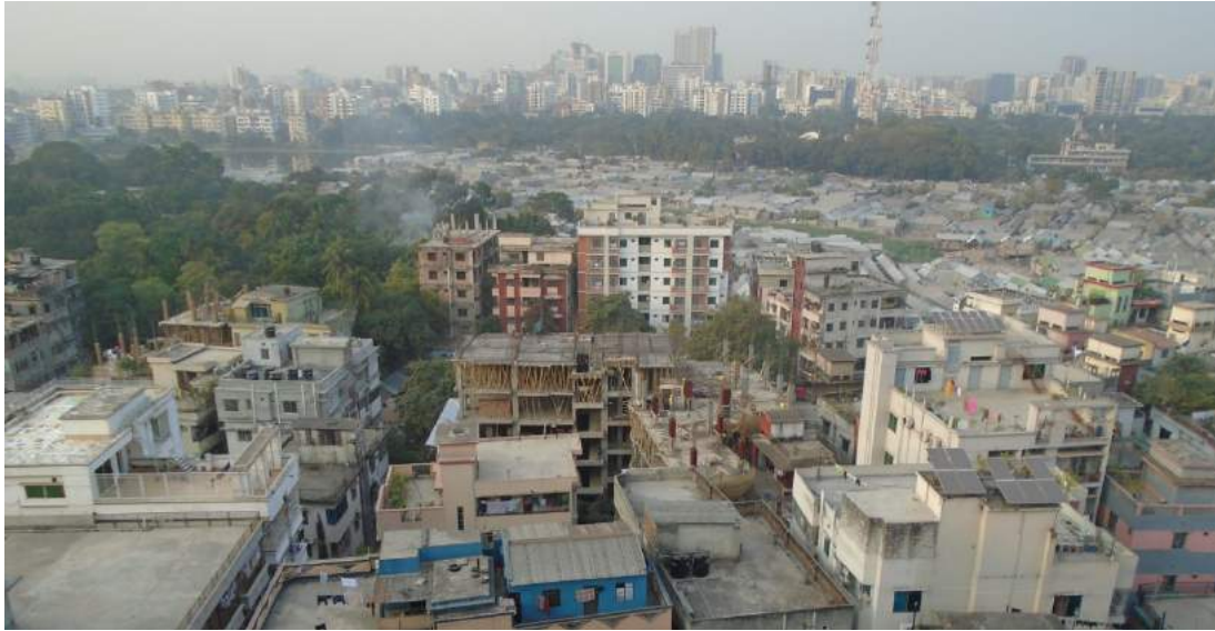
Figure 5.3: View from BRAC University: middle class high rise in the foreground, Korail slum beyond and the wealthy Banani and Gulshan districts in the distance (M Jones)
