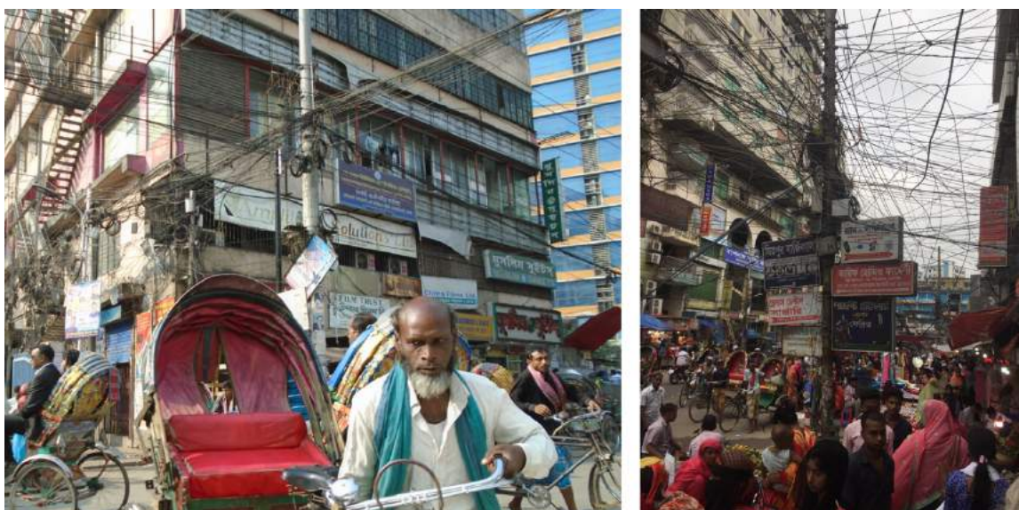
Figure 5.15: Street cabling in Dhaka (M Jones)
