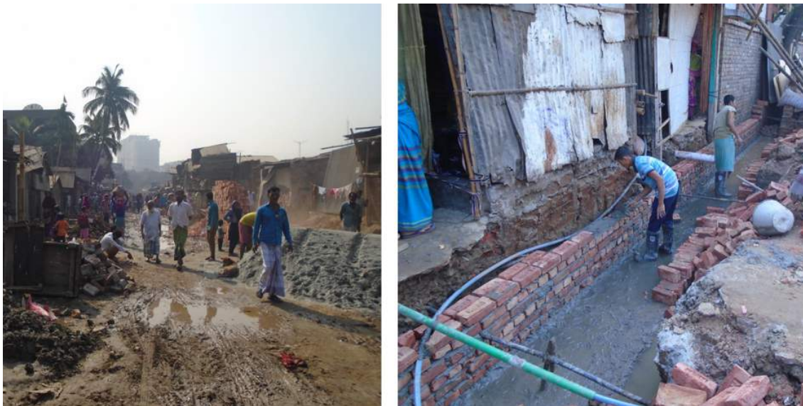
Figure 8.4: New road through KPB under construction on 22 January 2019 (M Jones)
