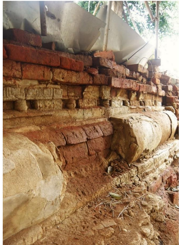
Figure 7.6 Architectural stucco enhancing the mouldings of the superstructure base, and producing baluster and foliate designs, at the recently-excavated Dhammasala chedi , Nakhon Pathom. Photograph: Author.
