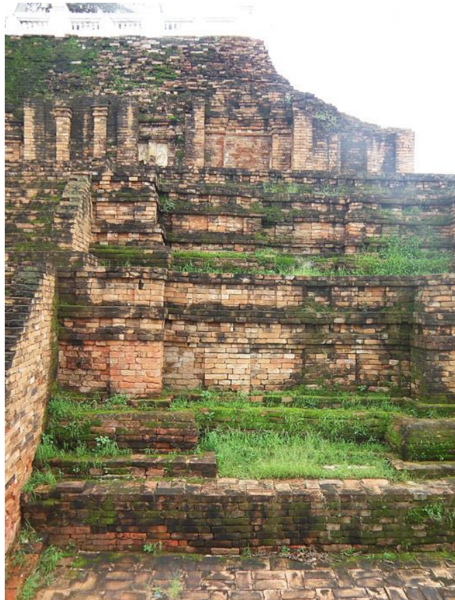
Figure 7.19 The three terrace walls at Phra Prathon Chedi, showing the multiple recesses per terrace. Photograph: Author.
