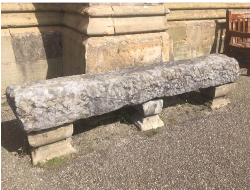
Fig 77: Fossiliferous marble stone located along south-side wall of Dunfermline Abbey Church. Note the different form of the supporting pedestal in the middle added to the two reported by Henderson (1879).
