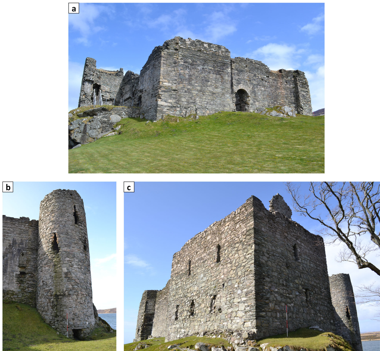
Fig. 4 a–c The main structural phases of Castle Sween. a Castle Sween from the southwest. Highlighting the sandstone-framed round arched main entrance and clasping buttresses of the primary phase enclosure; Romanesque features on which a c.1200 constructional date is based. The surviving upstanding sections of the otherwise collapsed secondary West Range and NW Tower are visible on the left of this image. No scale. b Castle Sween NW Tower from the north. Perceived architectural similarities between this circular garderobe tower and a feature at
