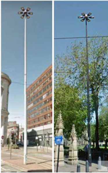
Fig. 13 Church Street streetlights
