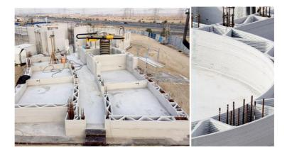
*Figure 2.* One can see reinforcement embedded conventionally in Dubai Municipality Building
