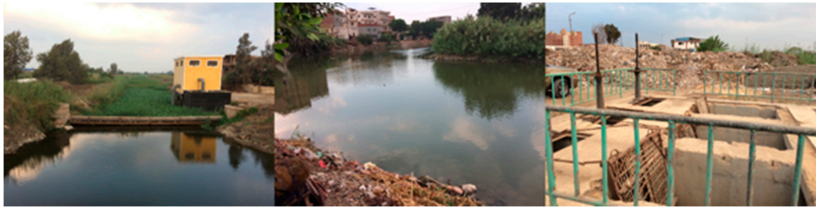
Figure 7. The pump station of Tilla drainage, Kased Canal, and the water plant in Tanta. Source: Author. Legend: The water in the drainage for pumping contains high level of eutrophication ( left ); the bank of canal is covered by solid waste ( middle ); the intake of the water plant is surrounded by garbage heaps ( right ). Location: at 31^{\circ}06'49.9'' N 30^{\circ}29'51.4'' E ( left ), 30^{\circ}47'02.9'' N 30^{\circ}58'24.0'' E ( middle ), and 30^{\circ}47'02.9'' N 30^{\circ}58'24.0'' E ( right ).
