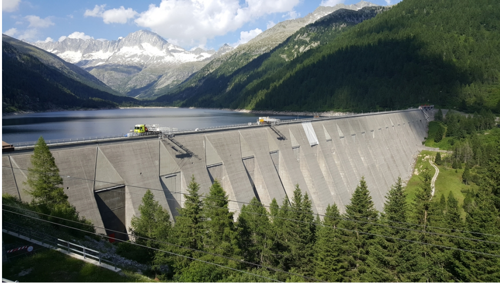
Figure 8. Cellular gravity dam (Marcello type) of Malga Bissina (photo taken by the authors on 05.07.2019).
